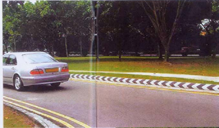
The new directional kerbs (inset) can even help to guide the direction of traffic flow.
