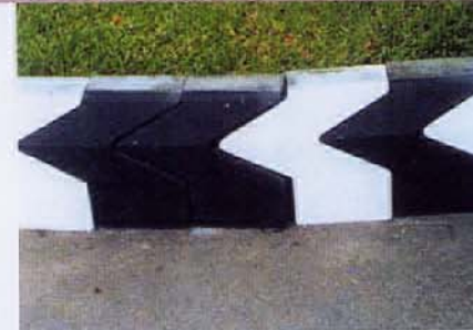
The new directional kerbs (inset) can even help to guide the direction of traffic flow.
