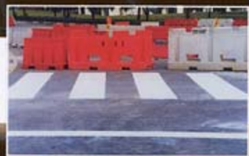
DAY VIEW: Reflective-mix Markings on bitumen surface
