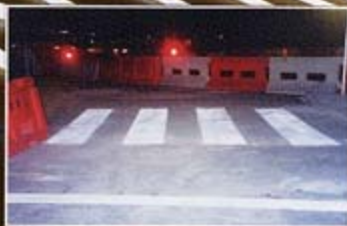
NIGHT VIEW: Reflective-mix Markings on bitumen surface
