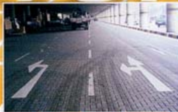
AFTER: Reflective-mix Markings on concrete block paver surface
