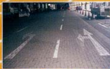
BEFORE: Thermoplastic/Paint markings on concrete block paver surface
