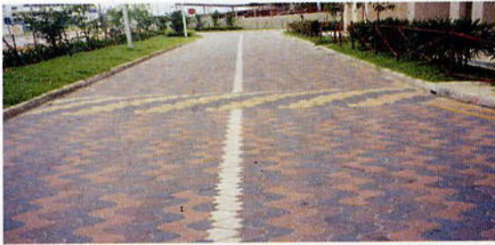
Fig. 6 HDB Road in Singapore, showing humped pedestrian crossing (HDB = Housing and Development Board of Singapore).
